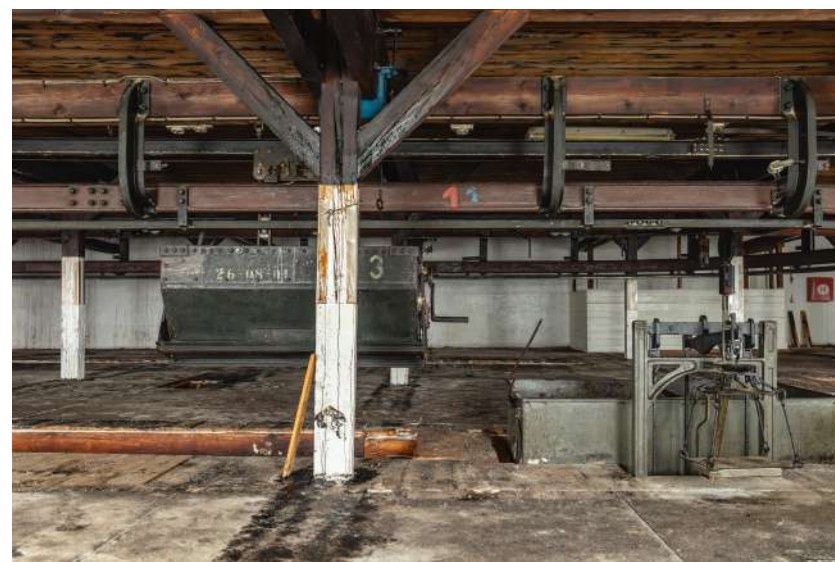
Sugar Warehouse with trolleys and a sugar weighing system.
